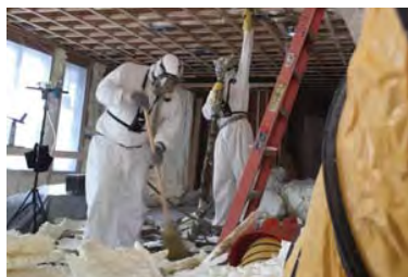
Workers applying SPF. PHOTO COURTESY OF RESEARCHERS AT UMASS LOWELL
