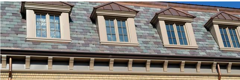
Four colors of Hilltop slate are carefully mixed to ensure proper distribution. The tiles are hand-nailed with copper nails in traditional style.
