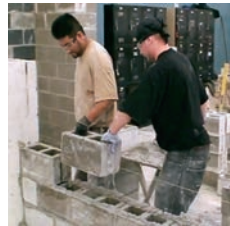
Workers use the two-mason lift technique to reduce stress of lifting and twisting.
