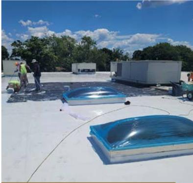
Local 97, Champaign, IL, roofers working for Top Quality Roofing apply LiquiTec over an EPDM fully adhered roof on a school in Gibson City, IL.
