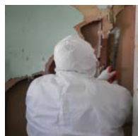
Worker wearing protective gear when removing mold.
