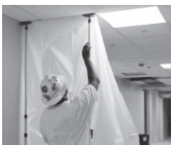
Worker establishing a containment area during an ICRA training class.
