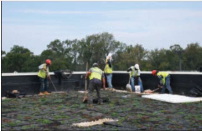
Local 30 crew put the final touches on the vegetative roof.
