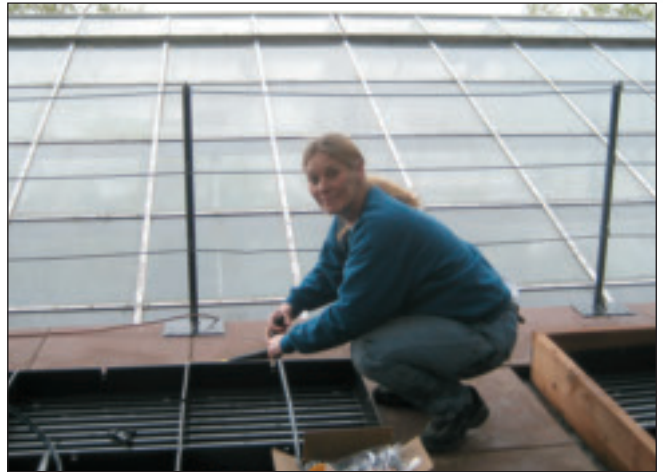
Jackie Maples works on the irrigation system.
