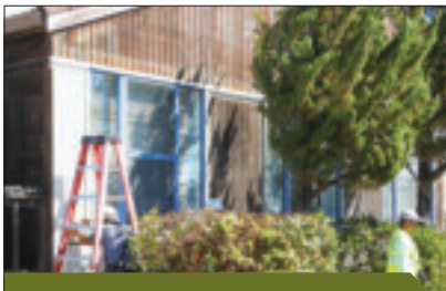
Local 81 roofers and waterproofer begin to install the new protective siding.
