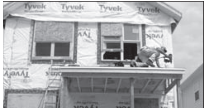
Local 65 Apprentice Nick Brzezinski of Robert Roofing nails down the shingles.
