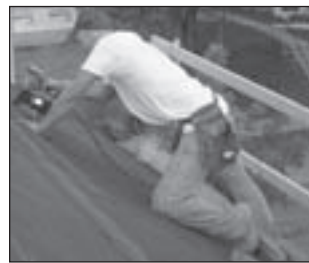
Local 65 Apprentice Ryan Monroe of Millen Roofing nails down the felt.
