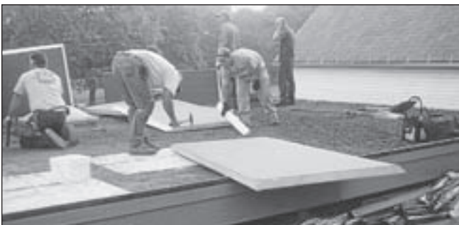
Local 134 volunteers preparing the roof deck prior to installing insulation.
