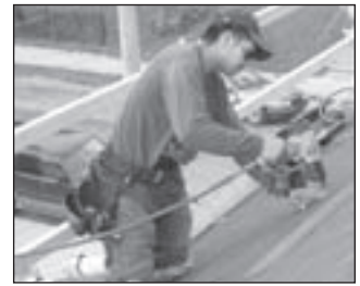
Local 65 Apprentice Ryan Monroe of Millen Roofing nails down the felt.
