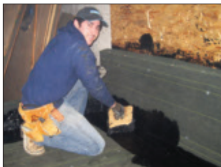
Apprentice Jesus Romo flashes a wall transition.
