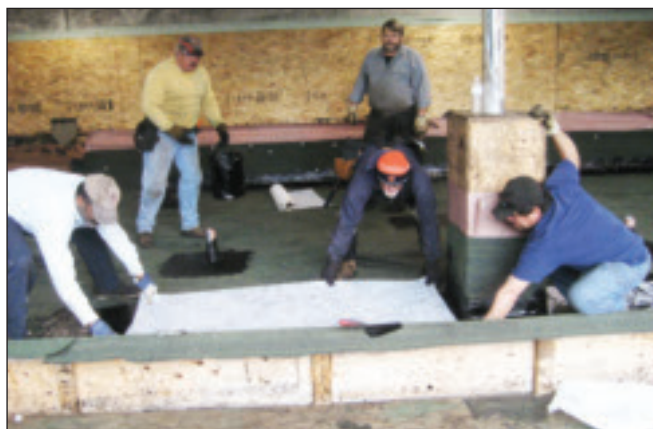
Journeymen Dave Hernandez (right), Phil Duffek (center) and Anthony Spires (left) lay the polyester sheet.
