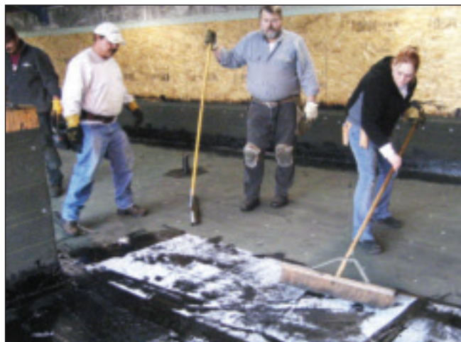
Apprentice Cassie Sikes (right) brooms the polyester sheet with instructor Steve Hurley (center) and apprentice Jose Talavera's (left) help.
