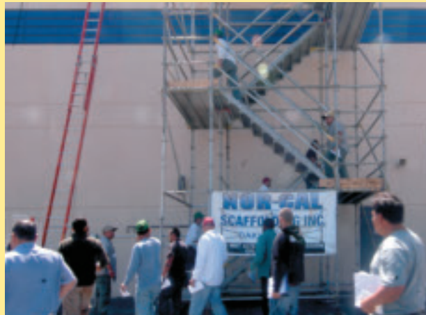
Stair tower by Nor-Cal of San Leandro, CA.
