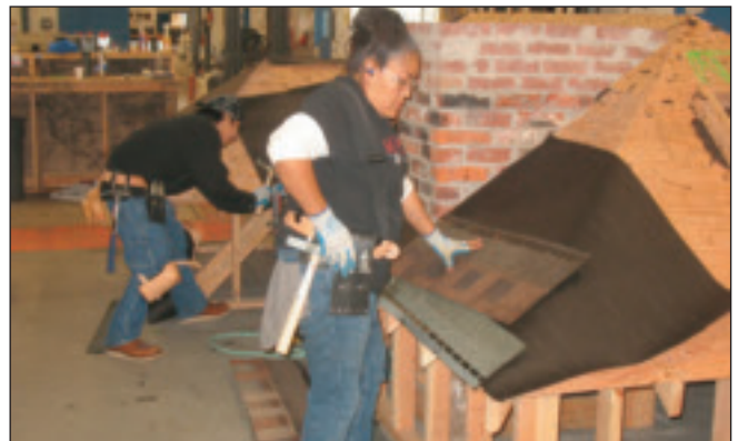
A RAPTOR student shingles on a mock-up.
