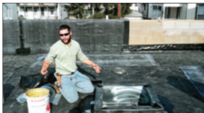
Tony Long flashes roof curb.
