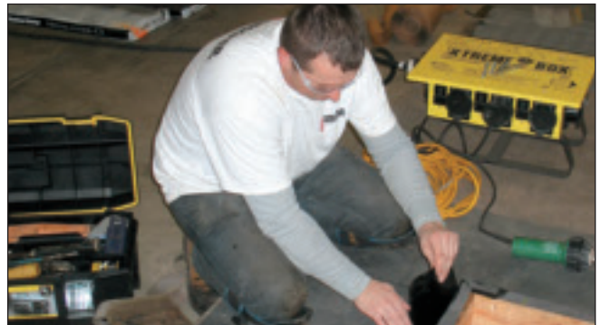
Second-year apprentice Ivan Medyanik wraps an EPDM corner in the single-ply/EPDM contest.
