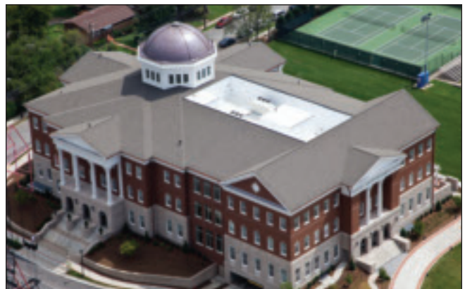
Signatory contractor Nashville Roofing & Sheet Metal installed a weatherproof copper dome for Belmont University's College of Law in Nashville, TN.
