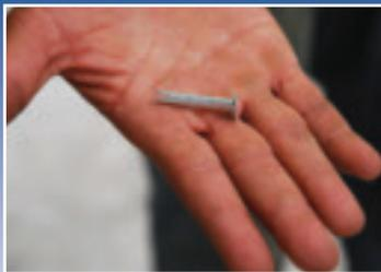
*The project required the use of special nails for the shingling. Instead of plywood, a gypsum substrate was used. The nails are barbed, and the end of the nail is divided so that it splits open when hammered, thus keeping the shingles from blowing off the gypsum substrate.*
