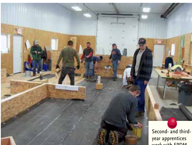
Apprentices Brian Bullinger and Nathan Brandt install wall flashings, while Nick Fader in the background wraps a curb.
