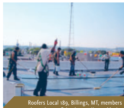
Local 189 members and initiates are at work on an EPDM roof in Billings, MT.
