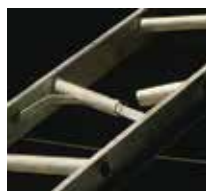
Not every defect is this obvious
