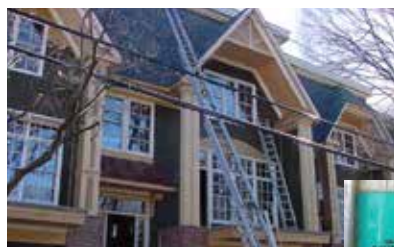
A painter was electrocuted when a metal ladder came in contact with a powerline.
