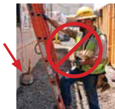
PHOTO COURTESY OF KIEWIT POWER CONSTRUCTORS
