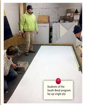
The enclosed area for single-ply hands-on training is equipped with a proper air circulation system for solvents and fumes.
