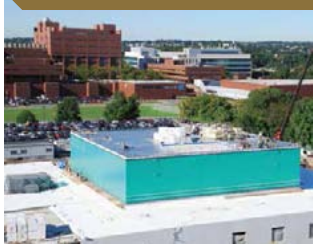
Roofers Local 33 members working for FMI Roofing roofed the Institute.
