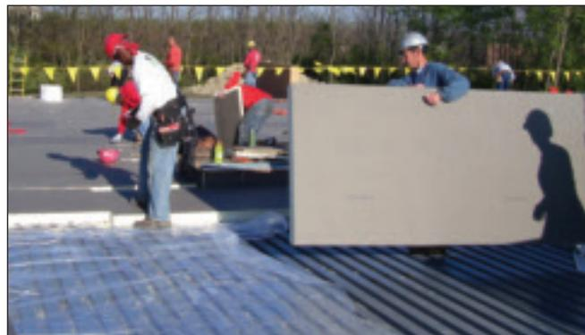
*Adding insulation in new roofs and retrofits is an exploding green roofing activity. Green installation of rigid insulation requires precise measuring and cutting.*
