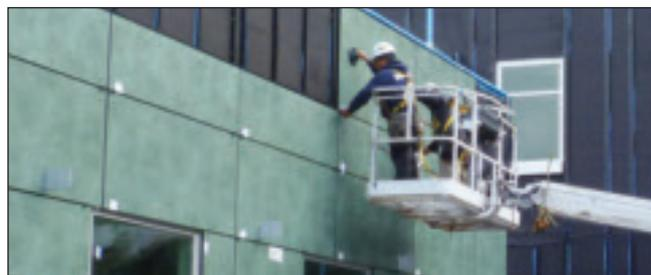
Exterior panels are placed over a green air/vapor barrier by Roofers Local 81 members on this new building at Marin College in the San Francisco Bay area. Roofers and waterproofers installed the air/vapor barrier and the panels, which are important parts of the green building envelope.
