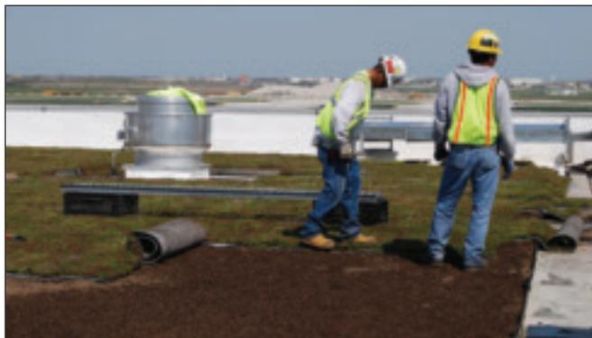
*Roofer's Local 11 members roll out plant mats on a new vegetative roof in the Chicago area. A vegetative roof is still a roof. So it is best installed by skilled union roofers.*
