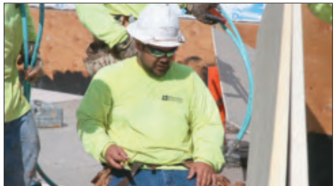
Sheldon Kahanaoi cuts insulation.
