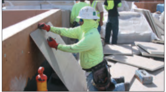
Clayton Rivera measures protection board.
