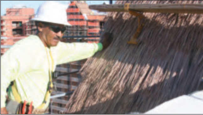
Venerando Aquino applies thatch.
