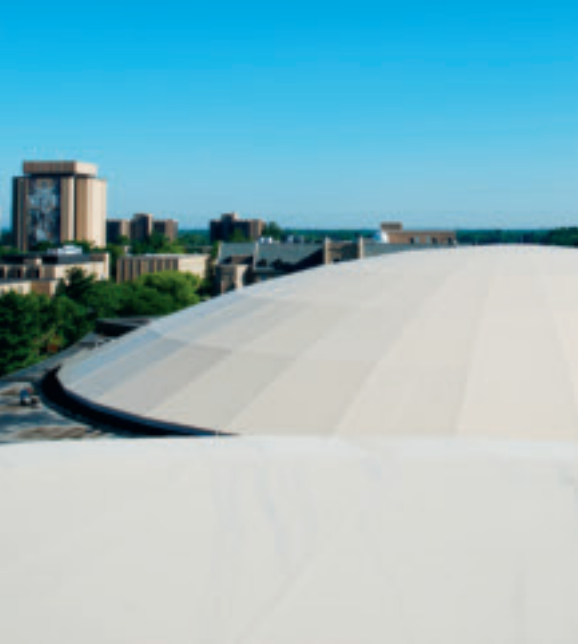
The finished north dome on the Joyce Center.
