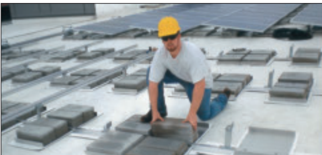
Laying the pavers that will support the PV system at GlaxoSmithKline.
