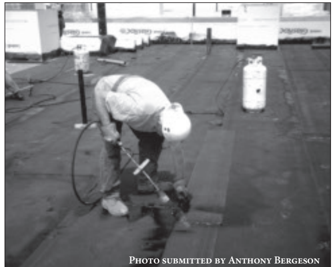
In the early stages, Local 54 roofers install a vapor barrier over DensDeck.
