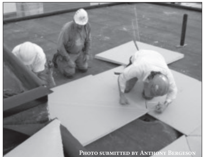
In the early stages, Local 54 roofers install a vapor barrier over DensDeck.
