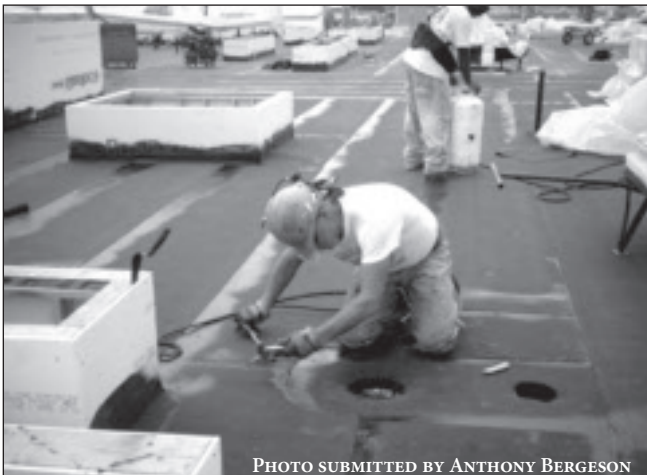
Chris Engberg prepares to detail a drain.
