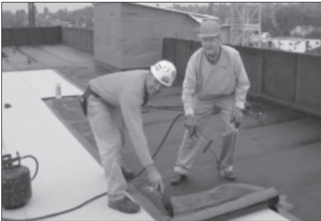
Foreman Anthony Bergeson and International President Kinsey Robinson apply torch down.
