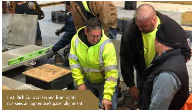
Chicago's apprenticeship facility has a large space devoted to training on paver systems.
