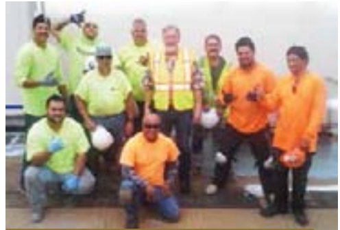
Beachside Roofing employees apply a Hydro-Stop system on the Queen's Medical Center in Honolulu. Kneeling: Chris Fuga and Ernesto Amian. Standing, left to right: Kawika Teixeira, Blake Nahinu, Claudio Aquino, Ramsey Teixeira, Int'l V.P. Doug Ziegler, Richard Kinoshita, Dustin Kekona-Gaspar and Ivan Pakele.
