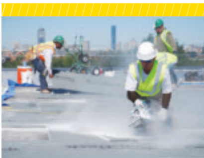
A Local 33 Roofer cuts the insulation to specifications.
