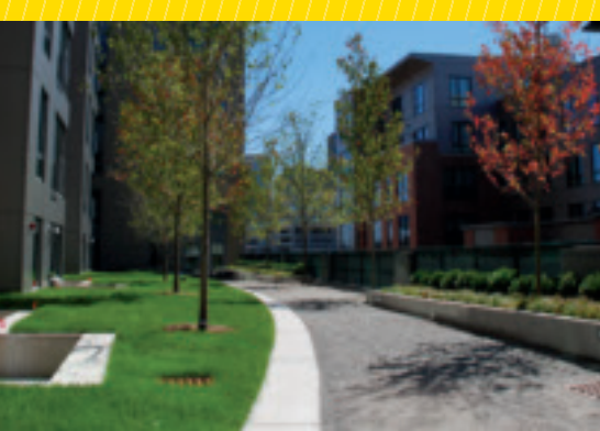
The fifth-floor terrace at The Victor provides private outdoor space for residents of the luxury rental development off Boston Harbor.
