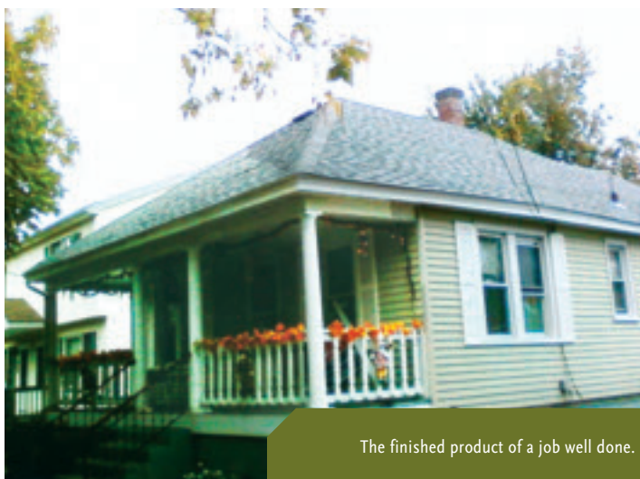
Homeowner Mary Forkey (center) is surrounded by Local 248 Roofers who re-roofed her home.
