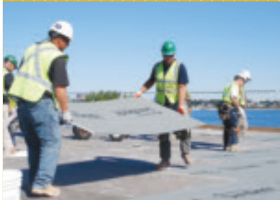
Laying the DensDeck on the Kennedy Institute.
