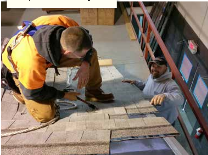
Local 149 apprentices on the advanced shingle mock-ups must tie-off while working.
