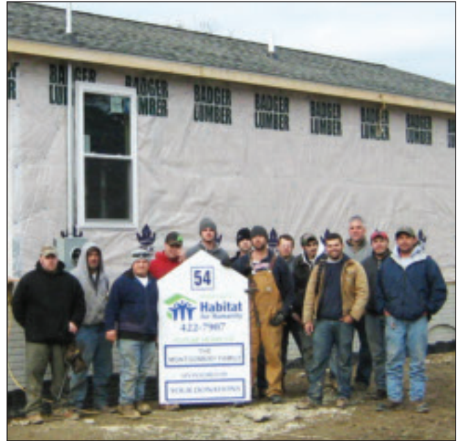
The crew of Local 242 roofers, proud of a beautiful job completed for Habitat for Humanity.
