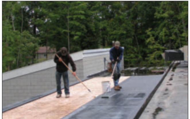
Local 23 apprentices prepare single-ply sheet.
