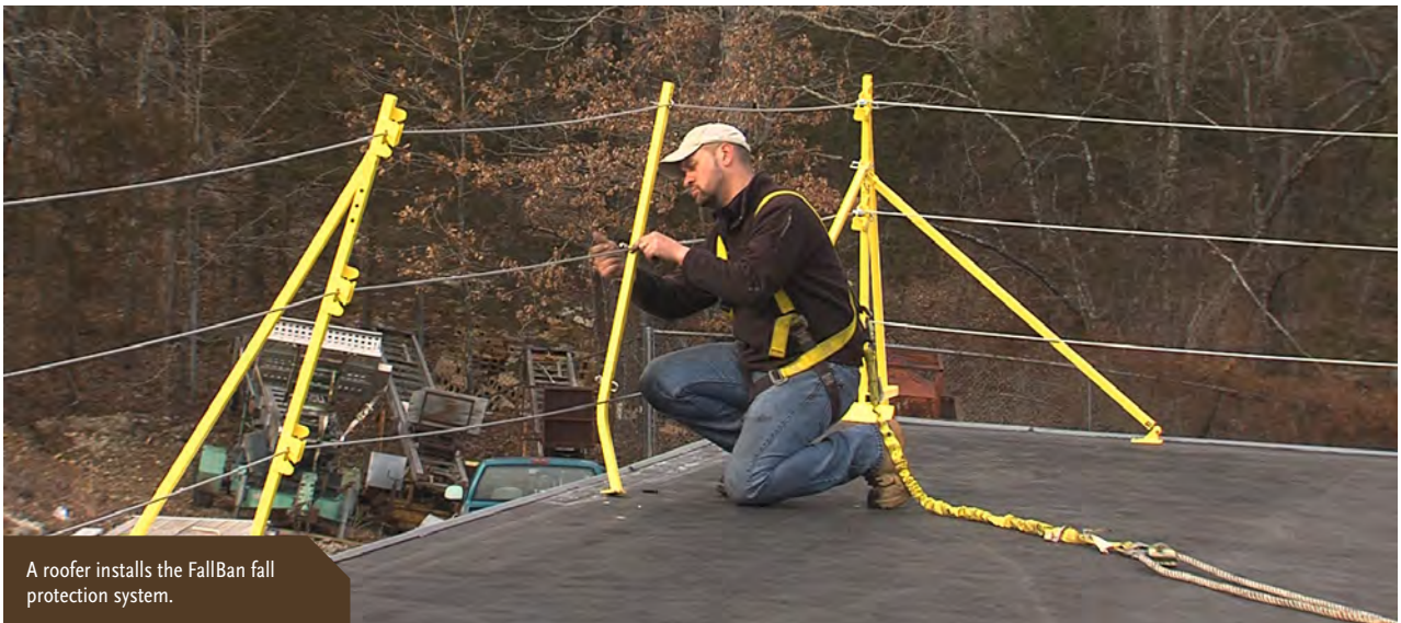
A roofing jobsite is outfitted with Ron Kempker's safety system.
