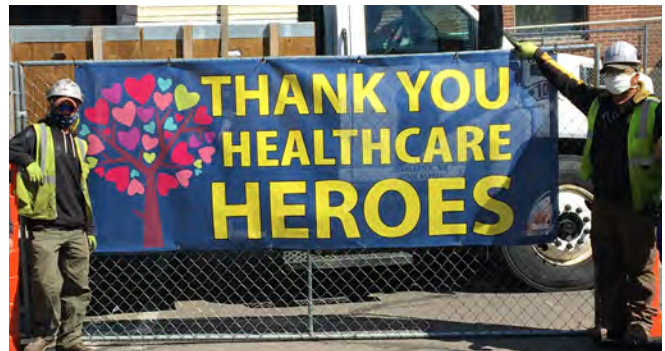
Local 96 roofers Shane Garb and Antonio Dominguez show support of healthcare workers while on their job site at Abbott Northwestern Hospital.
